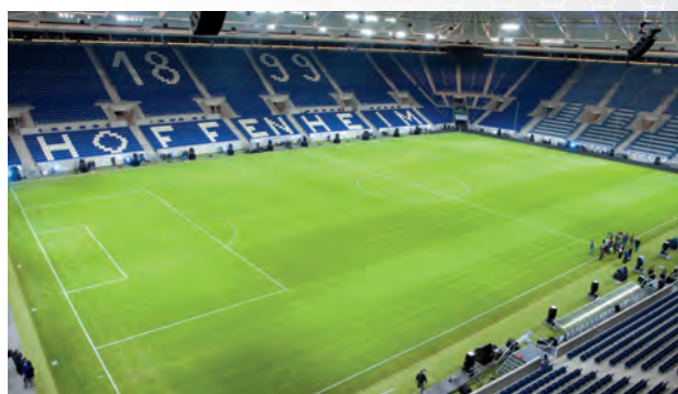
The roof structure of the football stadium belonging to TSG 1899 Hoffenheim mounted using LÖSOMAT cordless torque wrenches.
